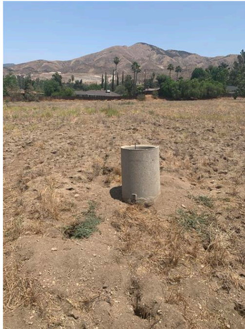
Photo #3 View of irrigation riser located in the central-eastern portion of the Property. View looking to the north.
